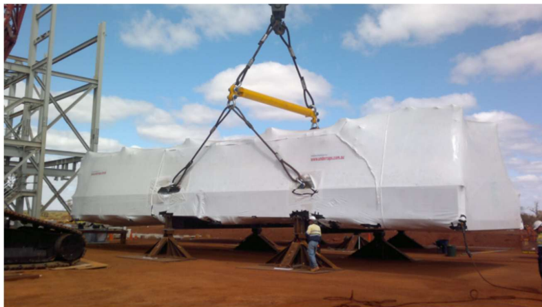
Figure 25: A view of FFP2512 being lifted
